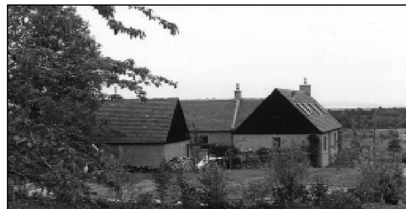
Pindlers Croft: New wing from the rear.
