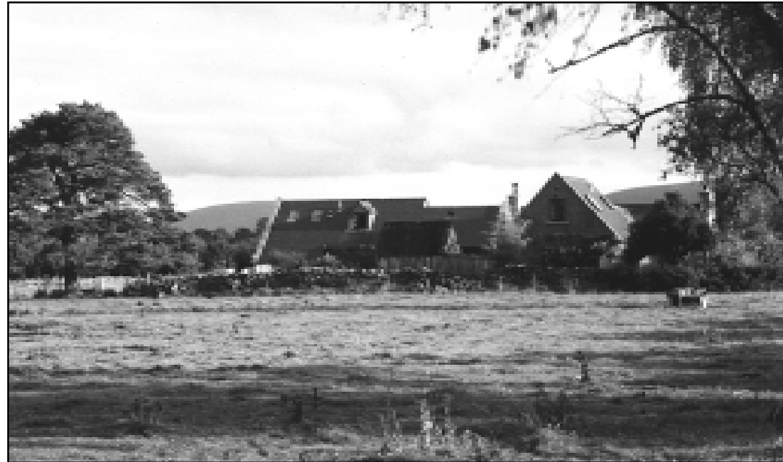
The renovation and extension of an existing croft cottage at Upper Knockando by Wittets of Elgin. A sensitive design using traditional forms and materials combine to create an attractive modern dwelling comfortable in its rural surroundings. The existing stone wall has been retained to visually anchor the house in the landscape.
